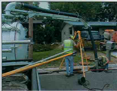
For ease of pump-out, access openings were located next to the curb.
